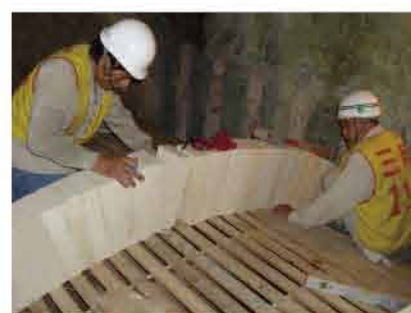
● 窯爐拱磚施工 Construction of furnace's arch bricks.
