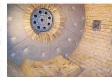
● 砌磚與搗固施工完成圖 Brick Installing and Ramming Constructure.
