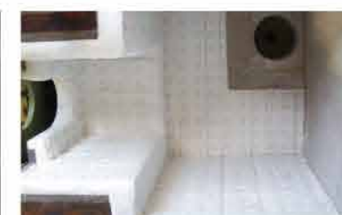
● 保溫材料施工 Construction of Insulating Material.
