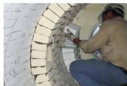
● 圓筒型窯爐施工 Construction of Cylinder furnace.
