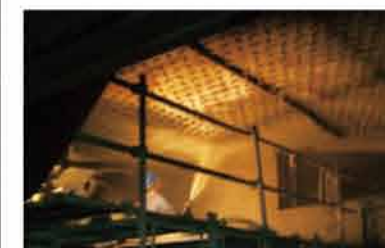
● 爐頂噴漿施工 The gunning of EAF Roof.
