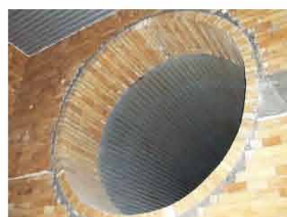
● 鋼鐵廠蓄熱塔施工 Construction of the heat accumulation Tower of Steel plant.
